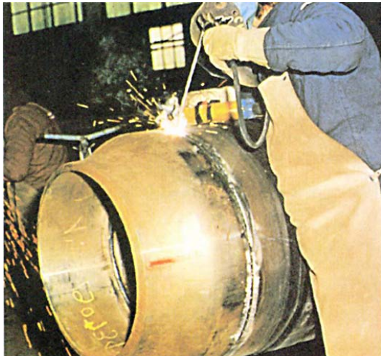
■ Welding of special joint
