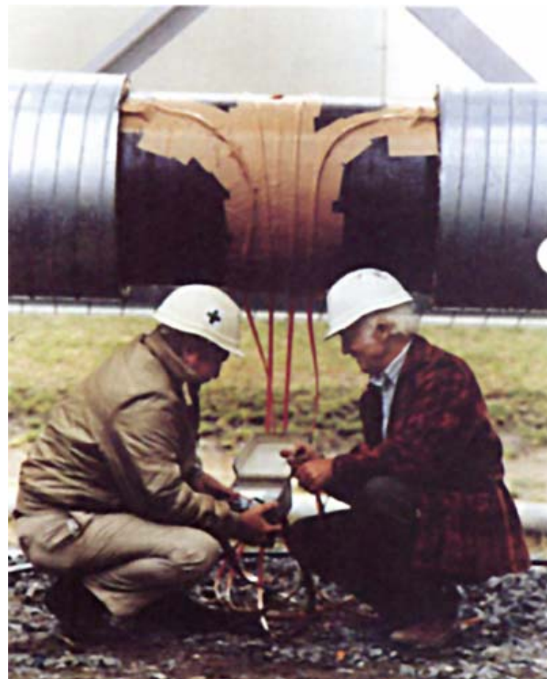
■ On site commissioning 600 nb systems. Site supervision in action
