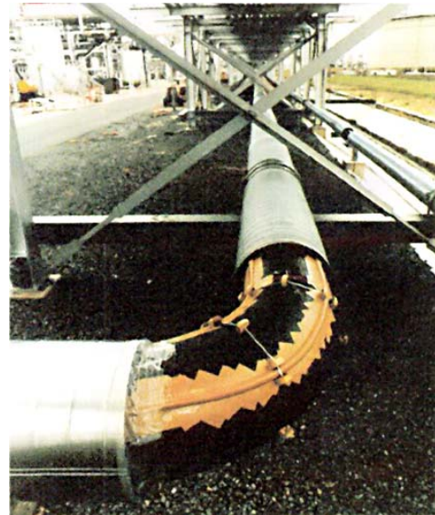
■ Heat tracing a site bend
