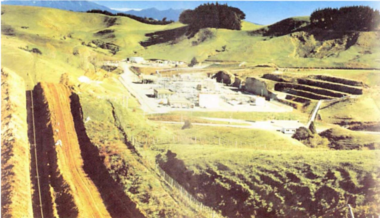
■ MiKee Field, Taranaki, New Zealand. Sixty km of heat traced HDPE jacket Insapipe flowlines connect 17 well heads to the primary separation station
