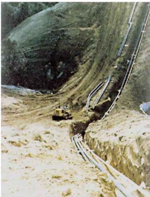
■ The process of jointing insaipipe involves welding, insulation and casing. It is simple, rapid and straightforward
